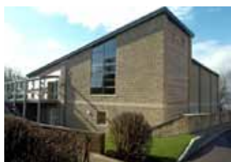
The Bradbury Centre, home of the hydrotherapy pool
